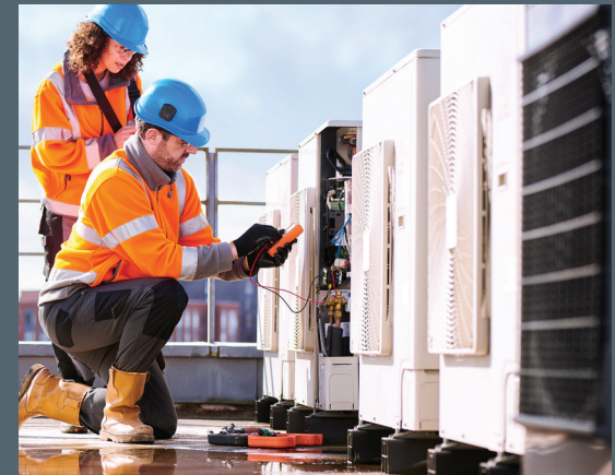
Installation and maintenance of air conditioning on the roof.
